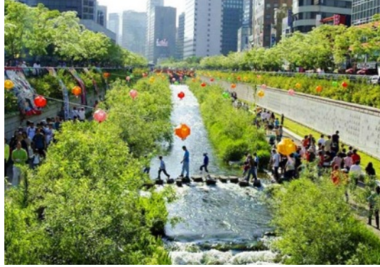
Figure 3. A gift to Seoul Citizens and the Ecosystem: Seoul conversion of elevated highway
